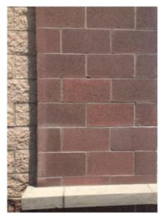
Designers should understand the appearance issues with smooth-face concrete masonry walls.
