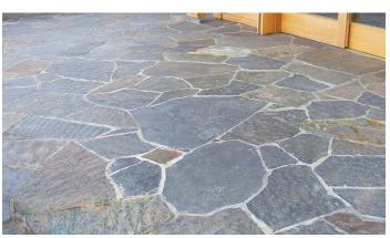
with a rubber mallet to level and provide consistent contact with the mortar bed. Compensate for the variations in the thickness by adding or removing mortar as you go. Try to keep your joint spaces about <sup>3</sup>/<sub>4</sub>" or so and avoid long, continuous joint lines.
