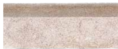
Indiana Limestone sill detail of face.
