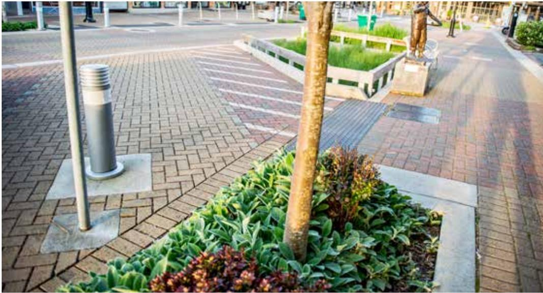
With its unique, patented interlocking spacer lugs, Eco-Priora® provides secure structural performance for permeable interlocking concrete pavements (PICP's). It works well under vehicular traffic, especially when compared to other "non-interlocking" permeable pavers.
