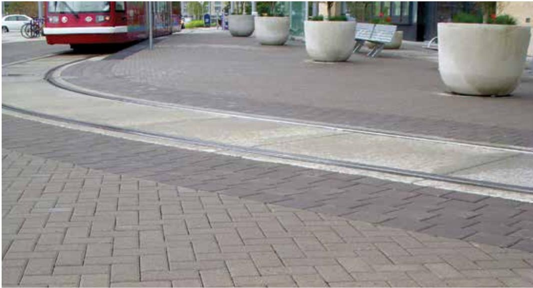
Holland 8 cm pavers offer the old-world charm of a simple brick shape combined with the renowned durability of interlocking concrete pavers. Simple in design, Holland 8 cm pavers are capable of meeting the demands of both architects and designers for a beautiful yet durable paving surface. Holland 8 cm pavers provide the additional structure needed for heavy-duty pavements.
