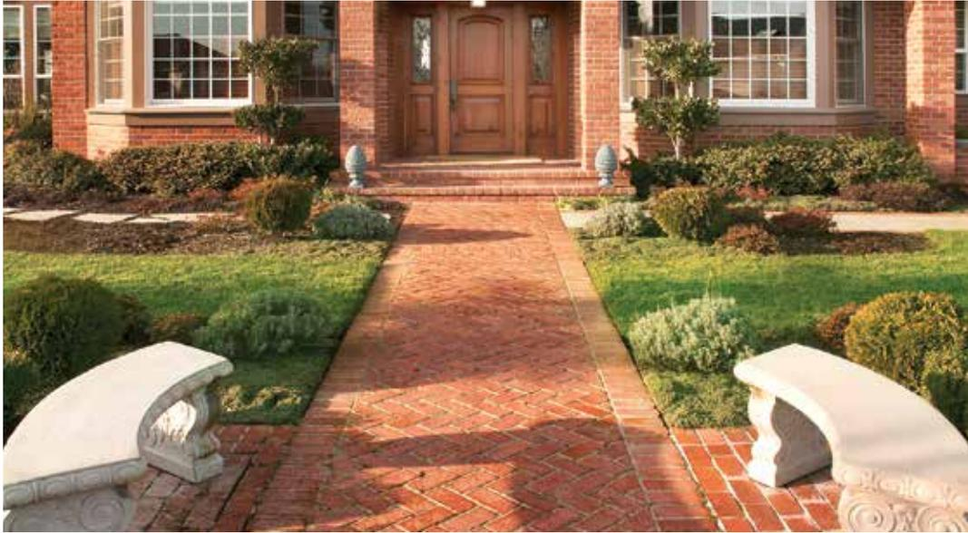
Clay pavers are designed to be set on a bed of sand over a crushed rock base. The net dimensions for width and length are 4x8 inches making it easy to lay them in a variety of patterns. Clay pavers can be set with the smooth or wire cut texture as the wearing surface and they permanently retain their natural color for lasting beauty.
