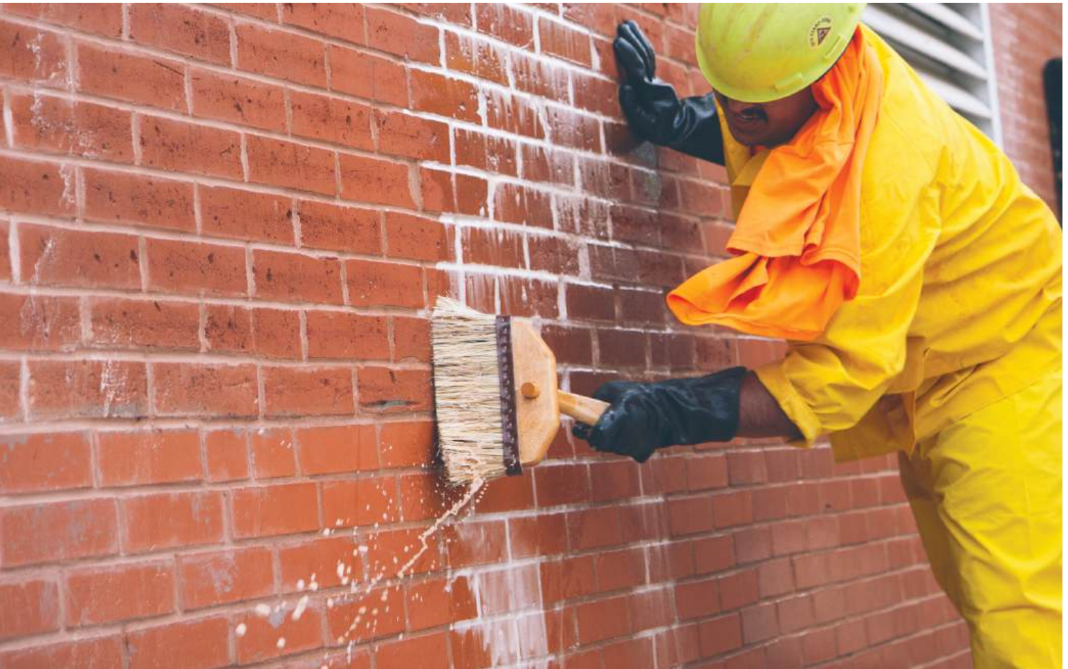
PICTURED: Cleaning brick with Prosoco® Sure Klean®
