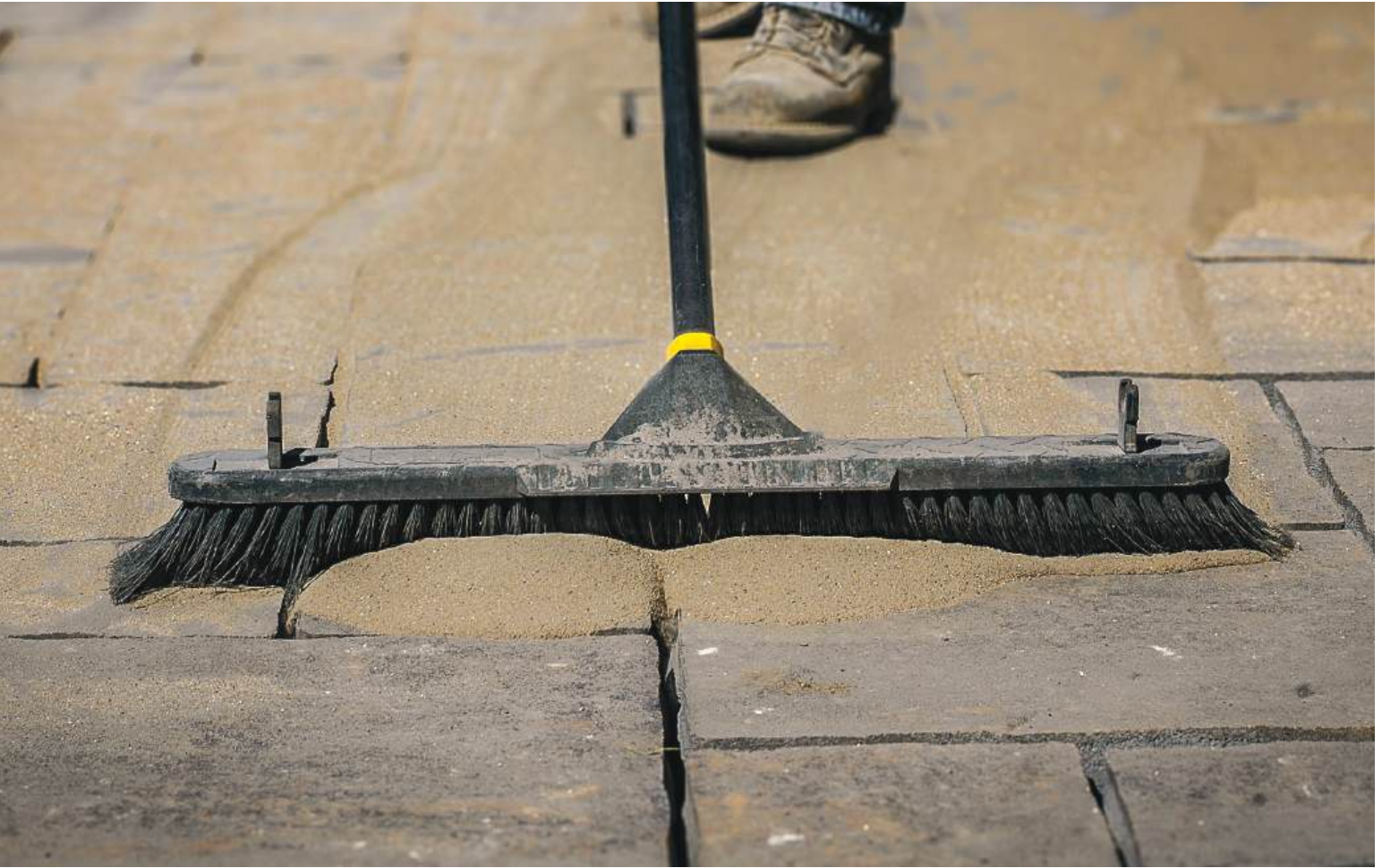
PICTURED: Filling paver joints with SEK-Surebond® Polysweep® X-Treme Wide Joint Polymeric Sand in Tan
