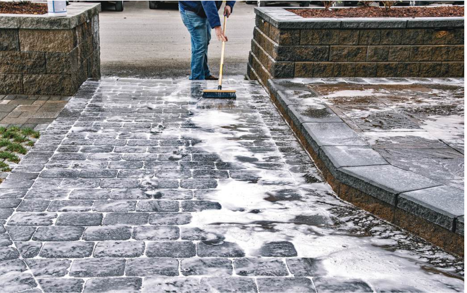
PICTURED: Cleaning Dominion™ pavers with Efflo Off
