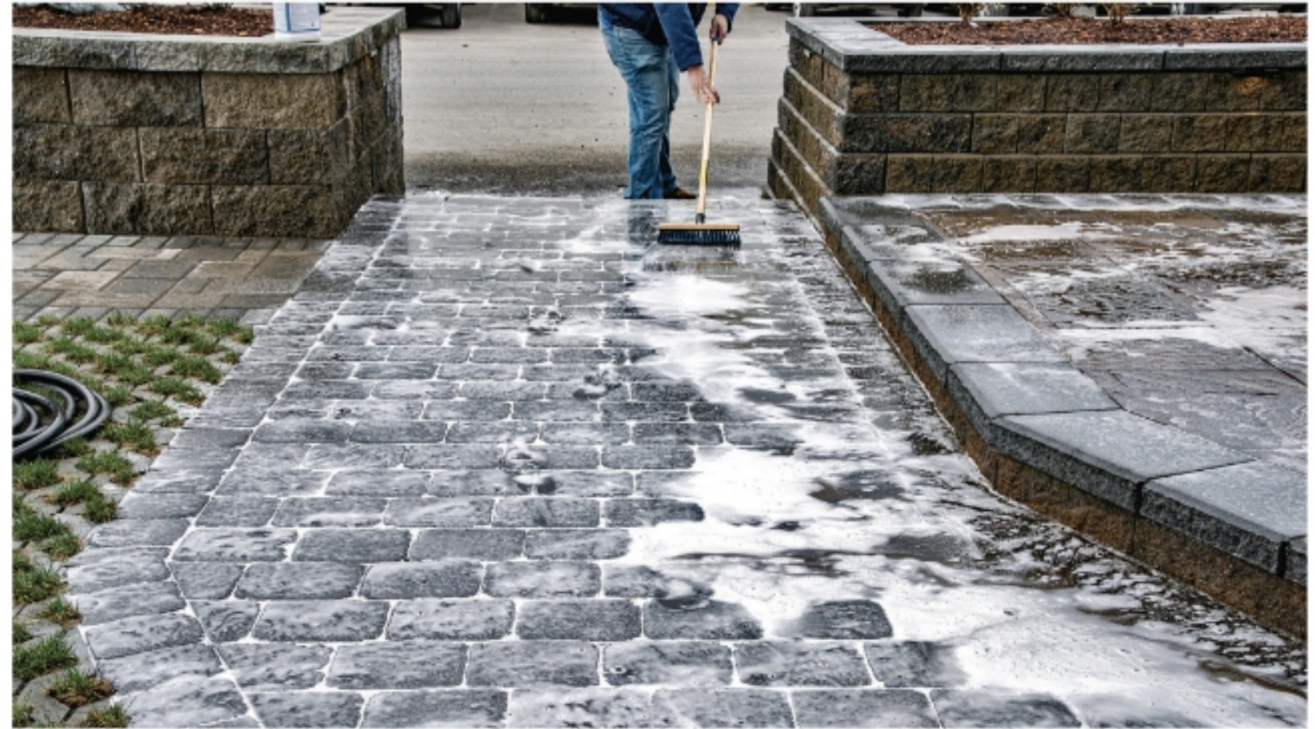
PICTURED: Cleaning Dominion™ pavers with Efflo Off
