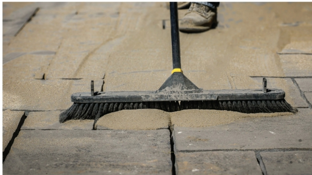
PICTURED: Filling paver joints with SEK Surebond® Polysweep® X-Treme Wide Joint Polymeric Sand In Tan
