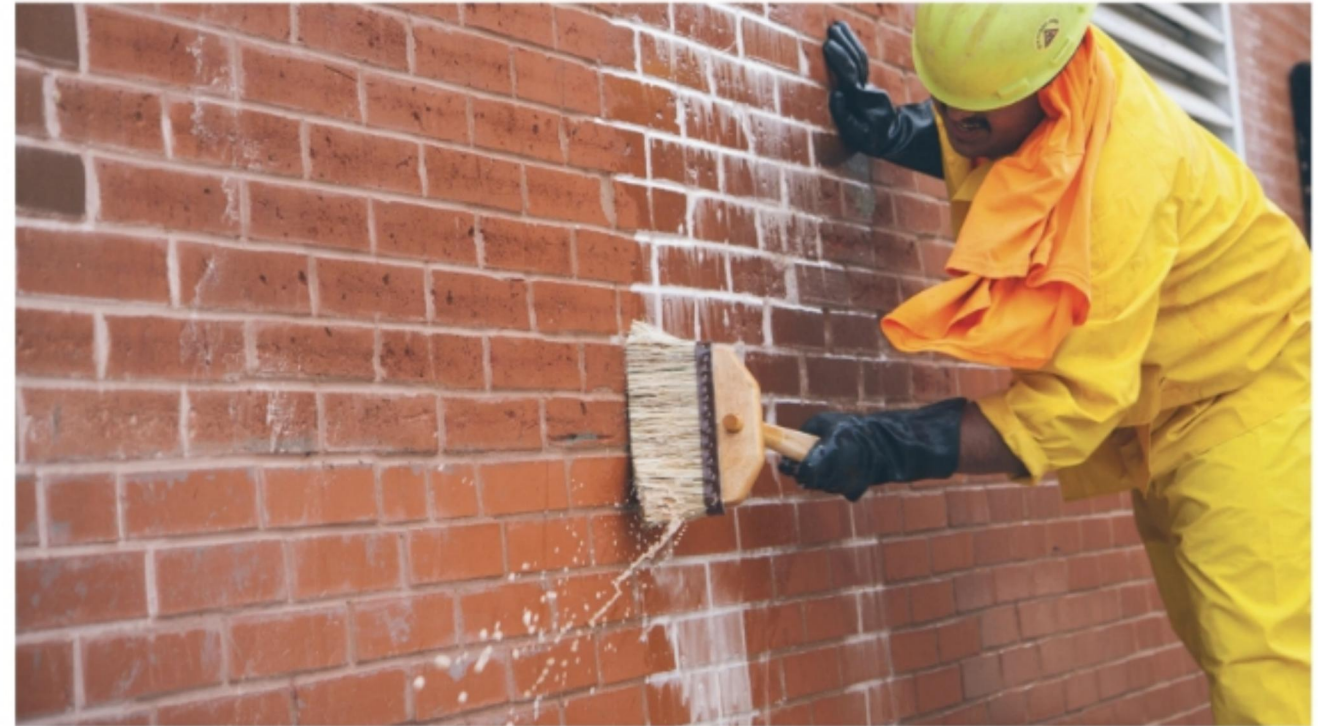
PICTURED: Cleaning brick with Proso® Sure Klean®
